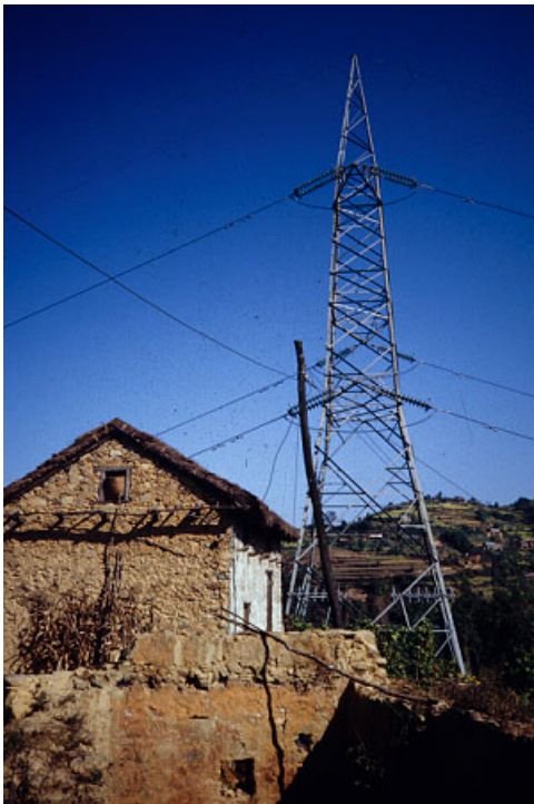
Figure 1: National Grid pylon and transmission lines which do not serve the local village where it is situated, on the Pokhara road, Nepal. Photo: Steve Fisher / Practical Action.
